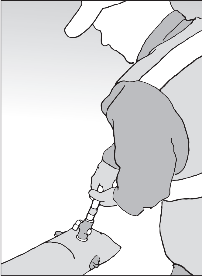
Figure 9 On extremely water sensitive sites, a 1" ball valve may be installed on drain port.
