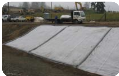
Hillside Covering for Erosion Protection
