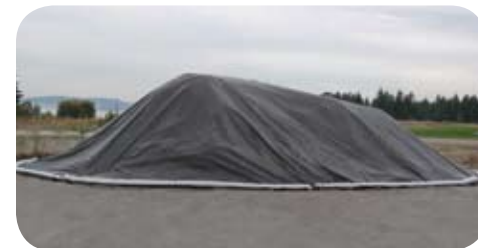
HazMat Spoil Pile Cover
