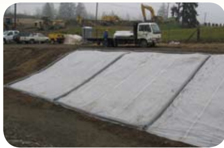
Hillside Covering for Erosion Protection
