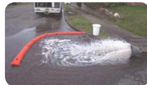
Water Diversion while Flushing Water-Line
