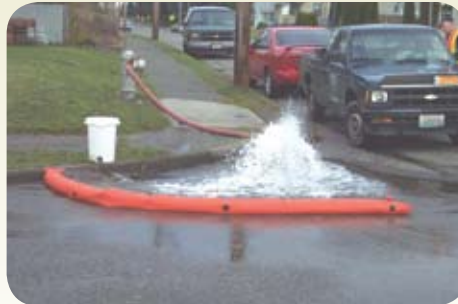
Safty Orange Ground Bladder Used for Water Control
